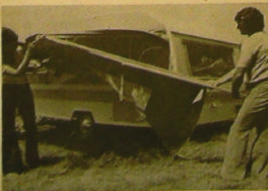
FIT THE SIDE WALLS (FEED IN FROM CENTRE OF RAFTER)
